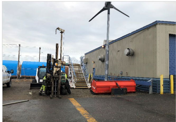
Exhibit 1-2: TWP installation at the former ARFF building
