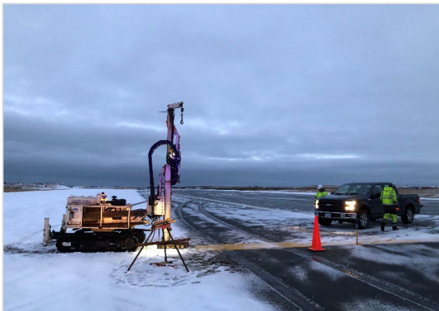
Exhibit 2-2: Drilling at the north end of Runway 3-21
